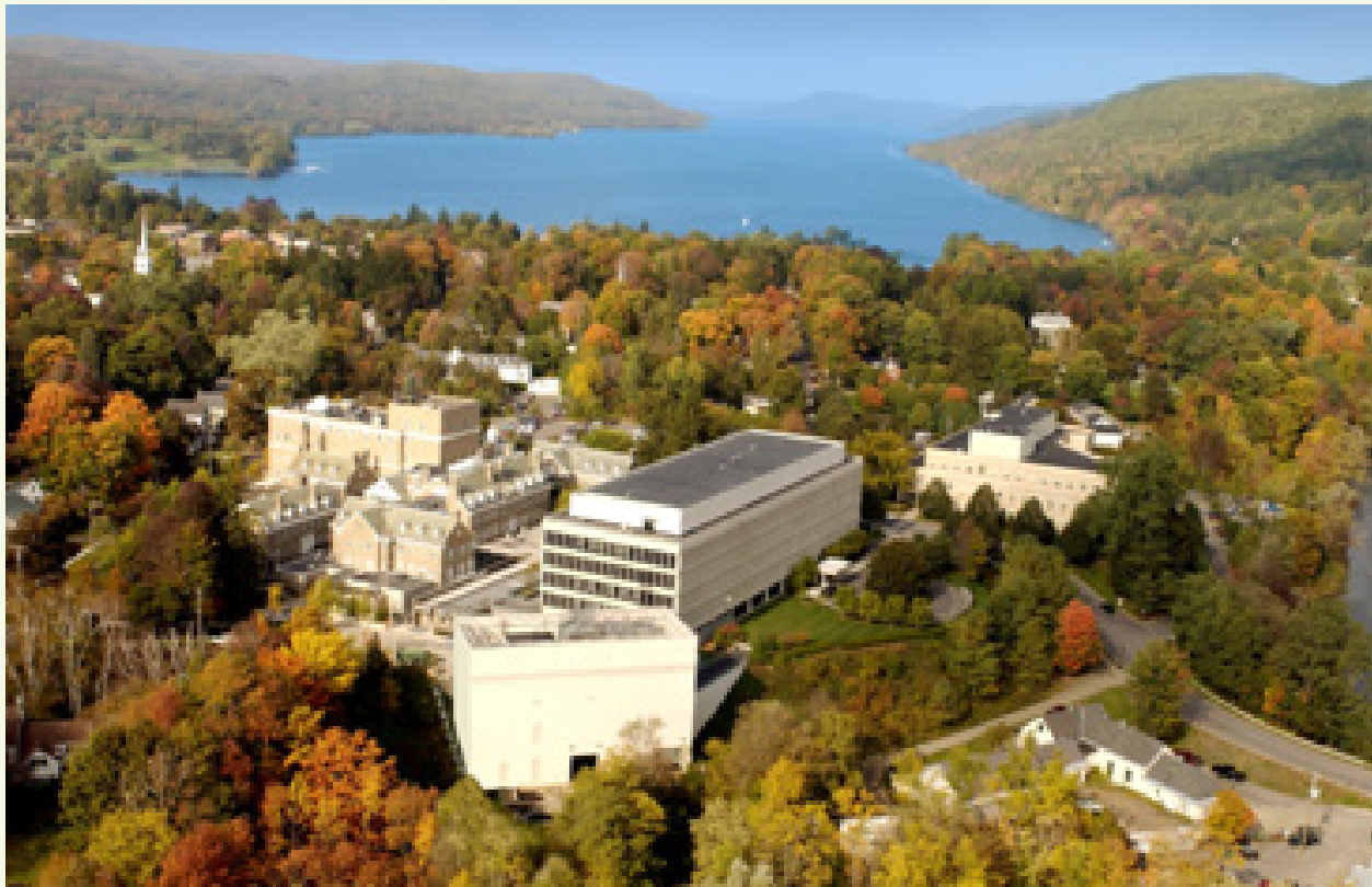
Bassett Hospital, Cooperstown, Otsego County
