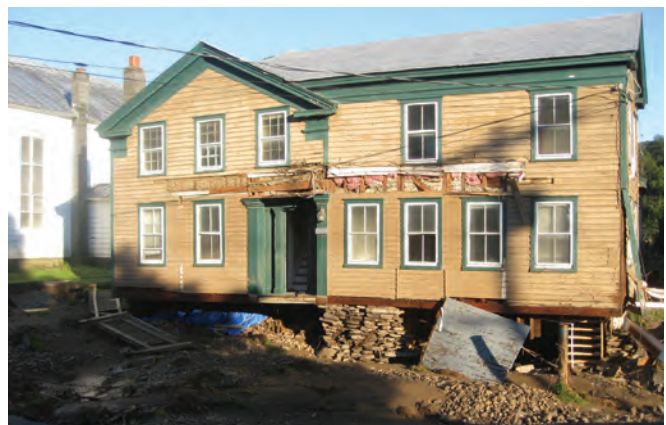
Flood damage ate away at this home's foundation. Photo is courtesy of Keith Graham.
