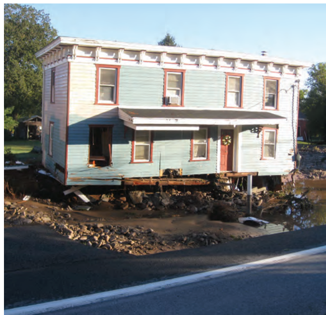
Home in Blenheim with washed-out foundation, missing siding and window. Photo is courtesy of Keith Graham.
