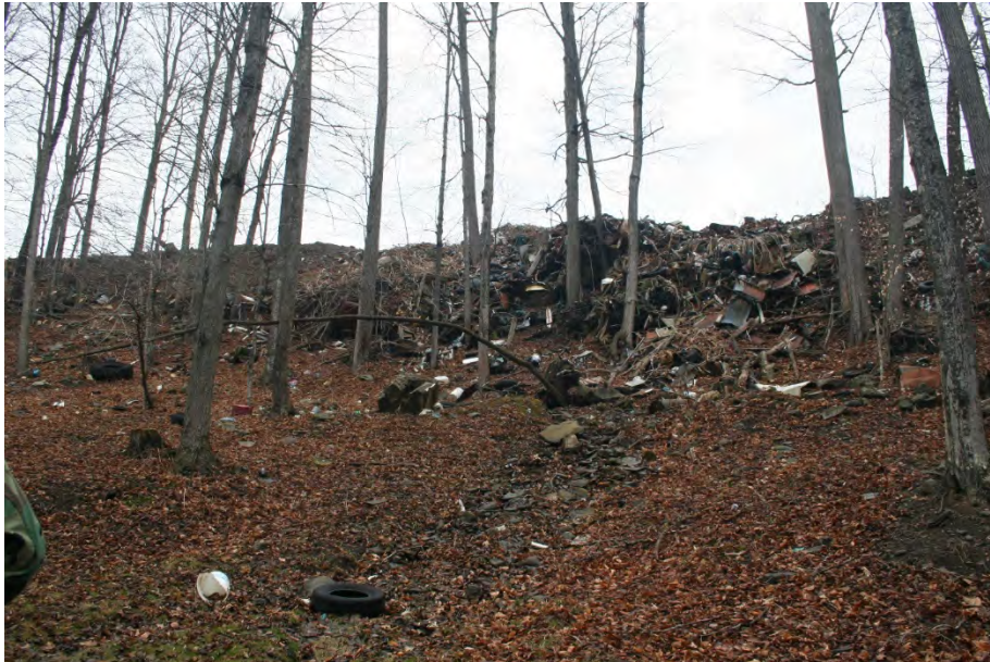
Main Branch at STA 40+00 Failing hillslope with farm debris March 7, 2017
