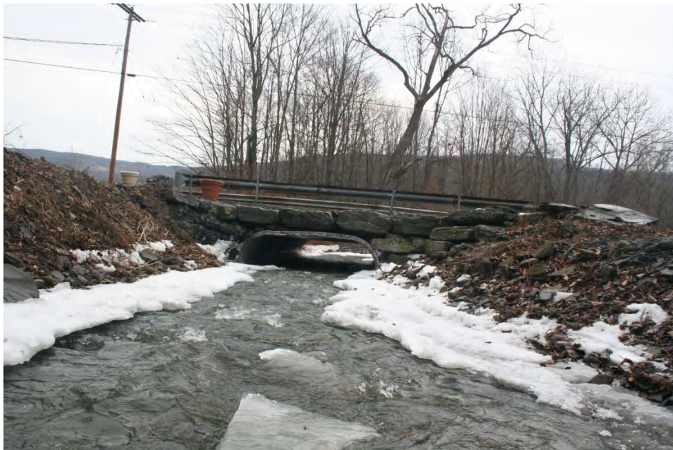
Main Branch at STA 12+00 Woods Road Culvert viewed from upstream March 7, 2017
