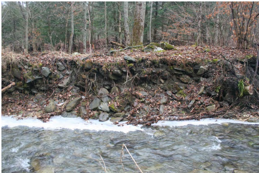
North Branch at STA 10+00 Channel incision March 7, 2017
