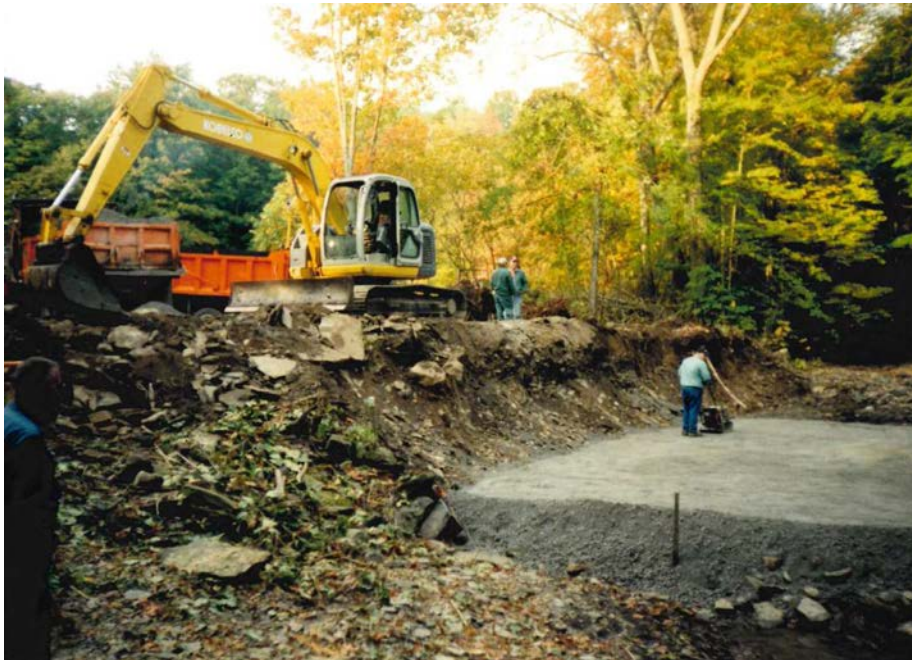
Figure 4-2 Existing culvert during construction
