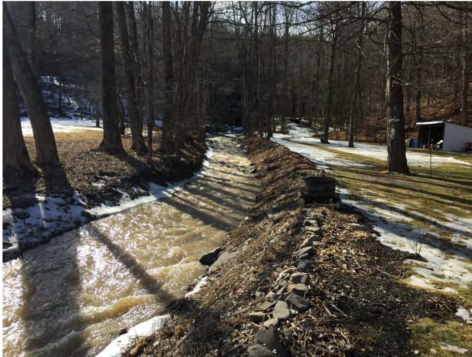
Main Branch at STA 12+00 Looking upstream from Woods Road Culvert February 24, 2017
