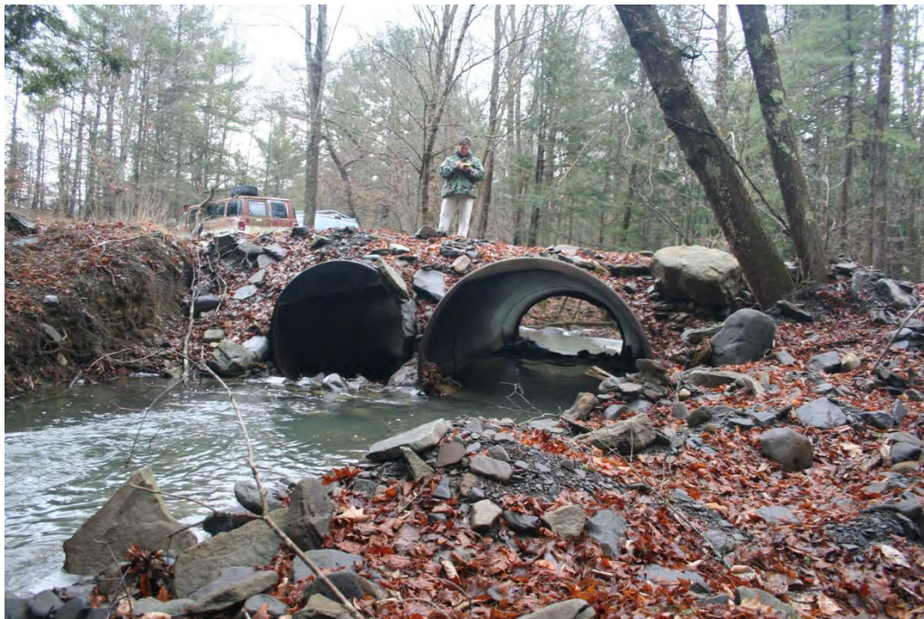
North Branch at STA 5+10 Channel crossing March 7, 2017
