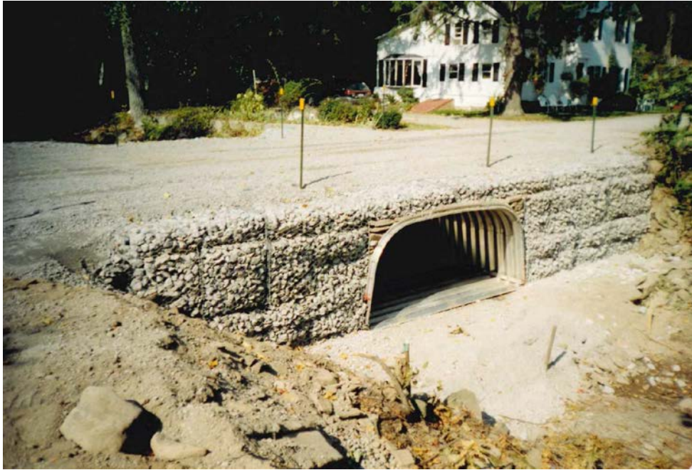
Figure 4-3 Existing culvert during construction, viewed from downstream
