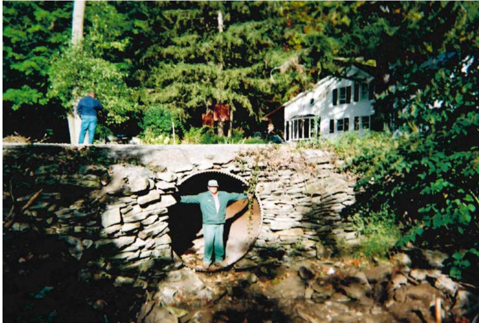
Figure 4-1 6-foot diameter round culvert that preceded existing culvert
