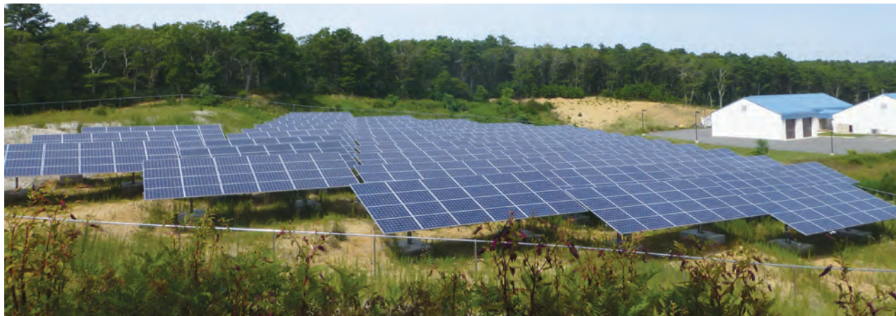
Figure 2.9. The 345.6 kW Brewster Community Solar Garden, located on a former municipal sand pit and dump site in Brewster, Massachusetts, provides enough electricity to power dozens of homes.
