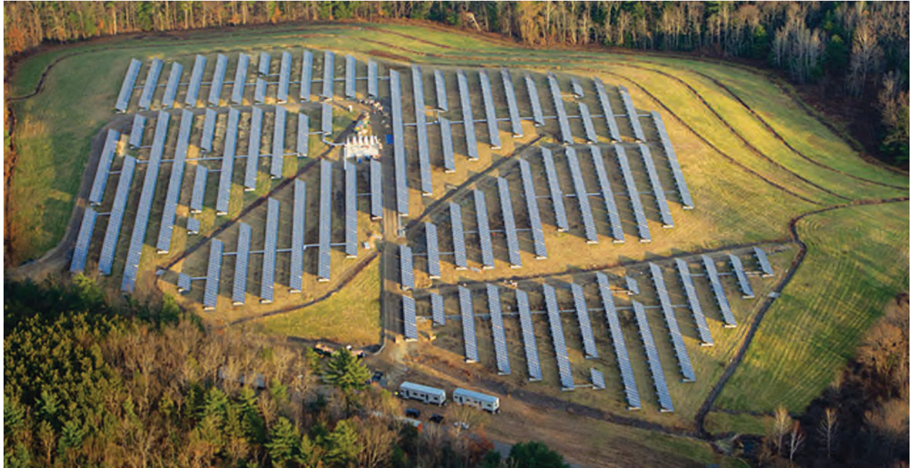
A 2.3 MW PV system on a capped landfill in Easthampton, Massachusetts
