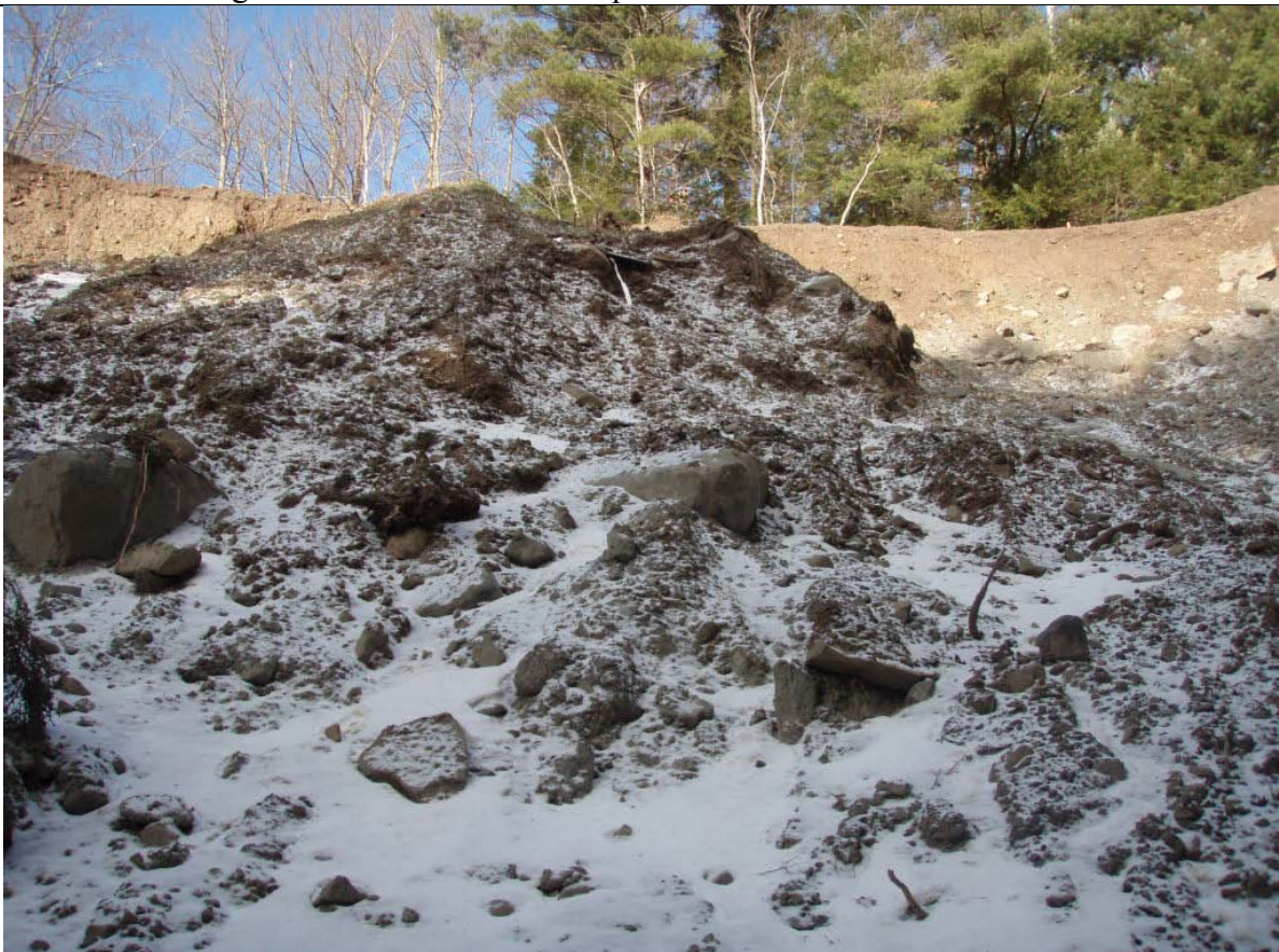
Photo 10: Looking N up at failed slope (approx. 55 feet high)
