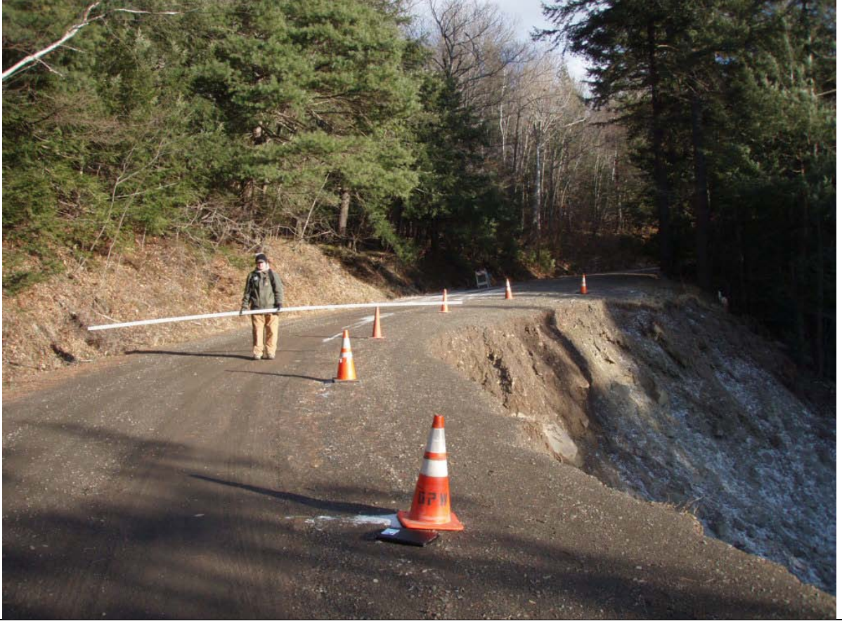
Photo 17: Looking East along town road damaged by slope failure
