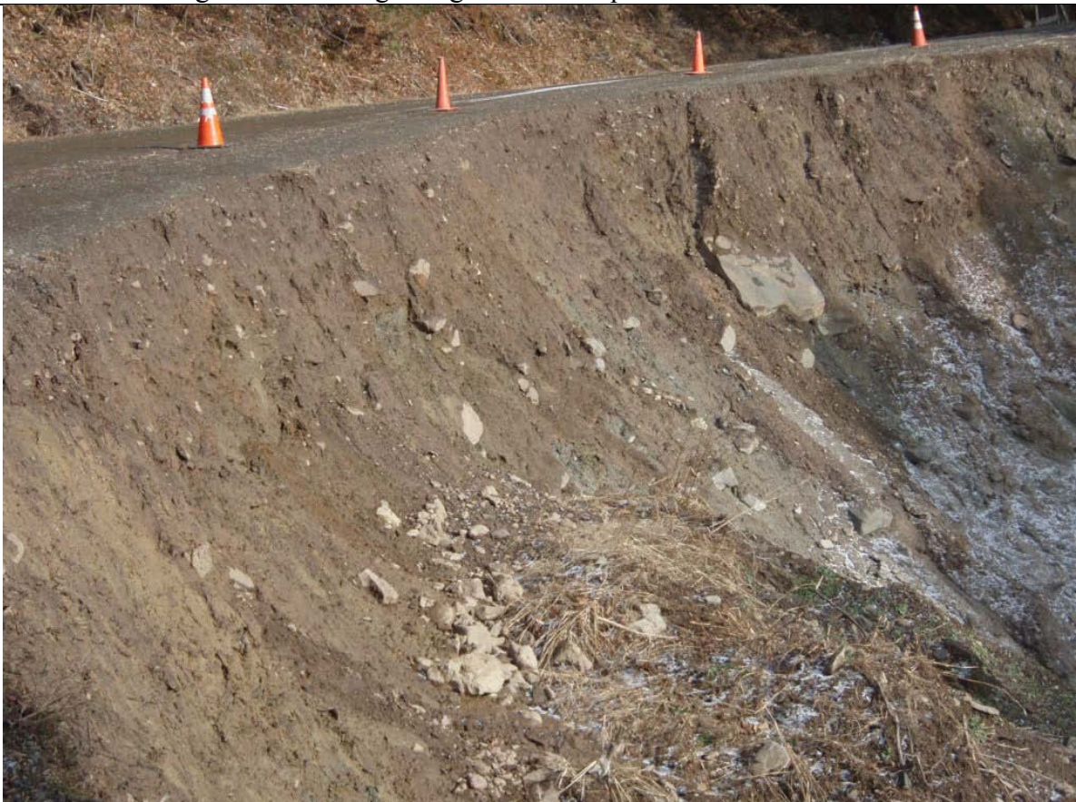
Photo 5: Looking East along slope failyure and damaged road
