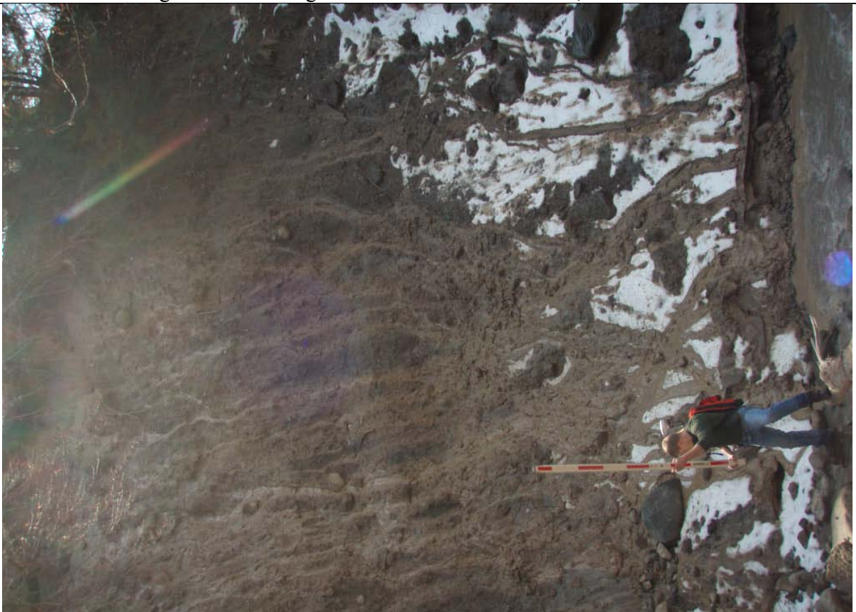
Photo 55: approx. 60-ft high raw left bank showing scarcity of armoring material
