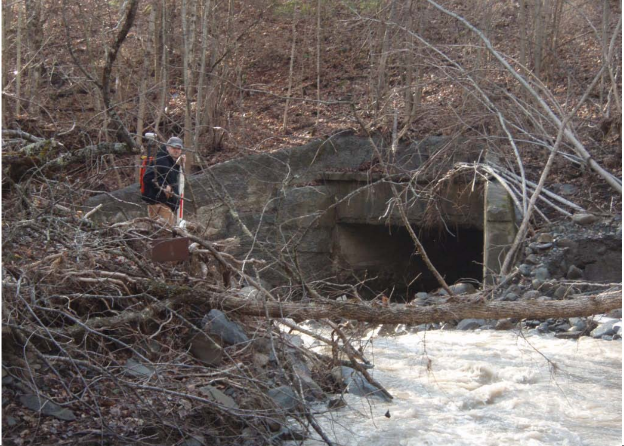
Photo 105: approx. 15'W x 7'H box culvert beneath Flat Creek Rd. (downstream end of reach)
