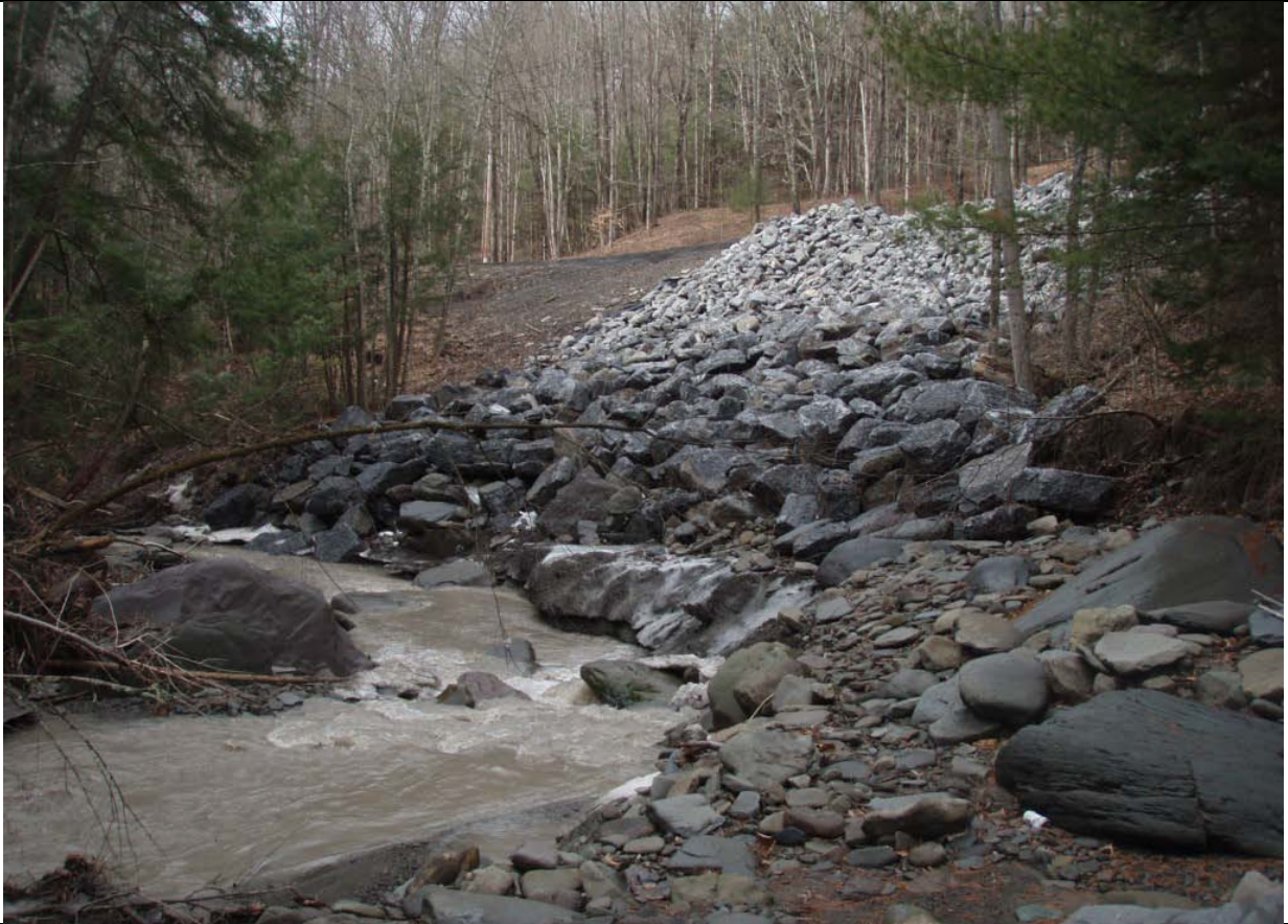
Photo 40: Looking DS at riprap slope installed post-flood to protect Flat Creek Rd.
