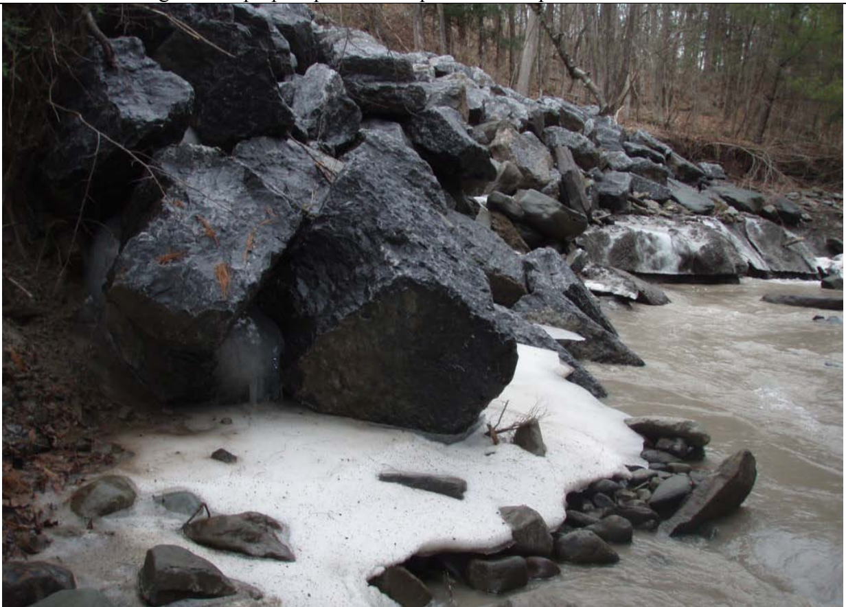
Photo 46: Bottom of riprap showing lack of toe key and resulting instability
