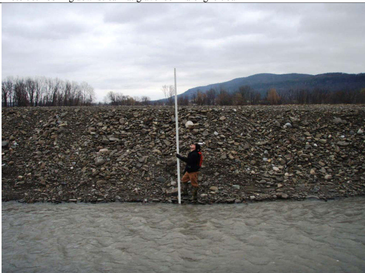
Photo 83: Looking across channel at ~ 8-9 foot high loose gravel berm on right bank
