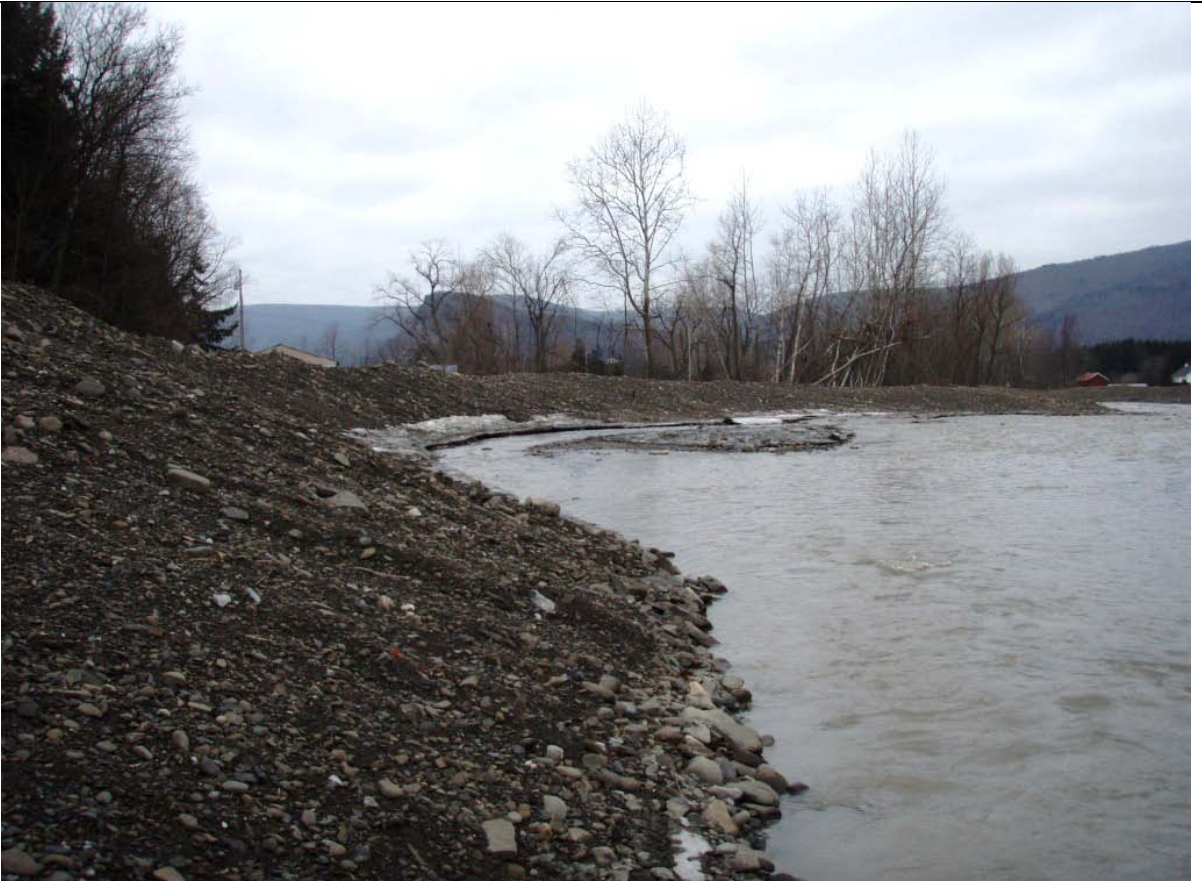
Photo 46: looking downstream at overwidened channel with high gravel berm on left bank
