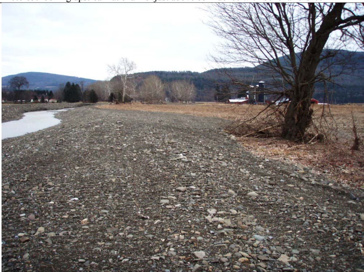
Photo 94: looking upstream at gravel berm along left bank of channel & floodplain
