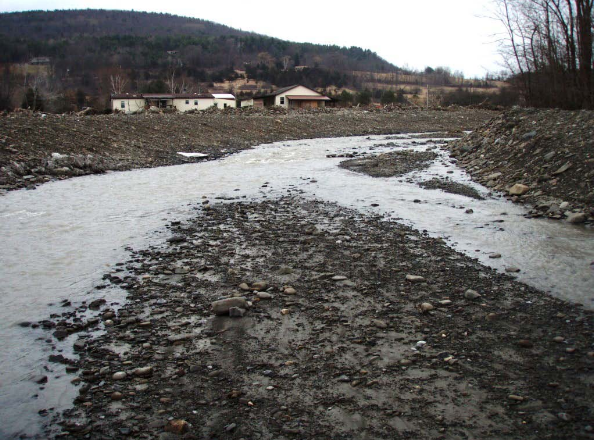
Photo 25: looking upstream at overwidened channel with loose gravel berms on both banks
