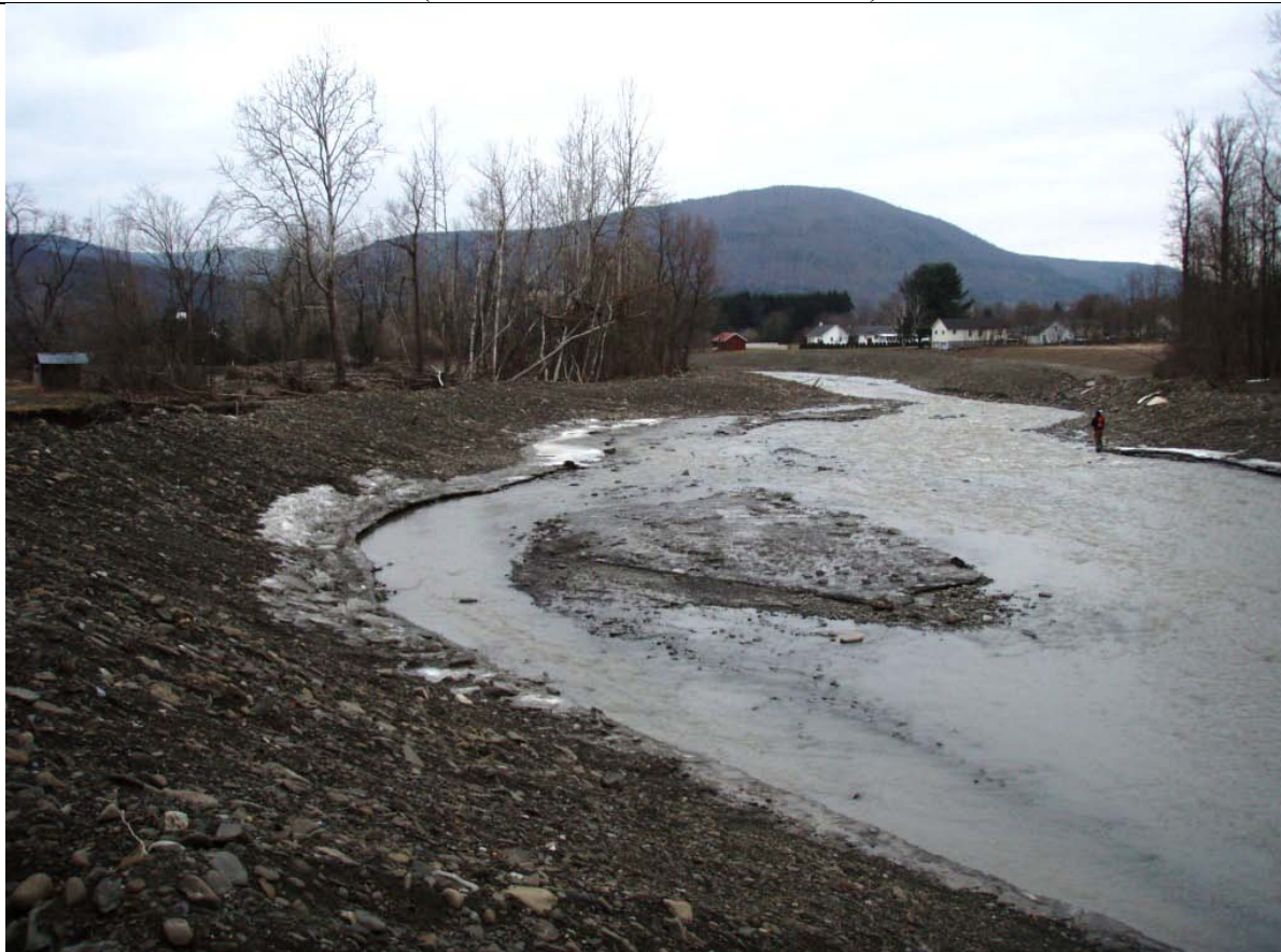
Photo 50: looking downstream at overwidened channel with high gravel berms on both banks
