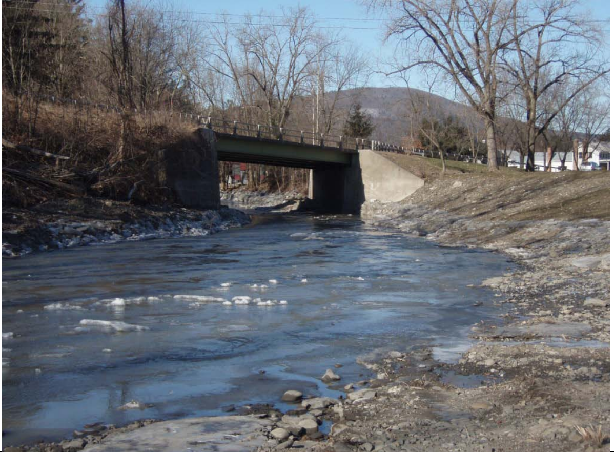
Photo 2: Looking downstream at NYS Rte. 145 bridge as DS end of Reach B
