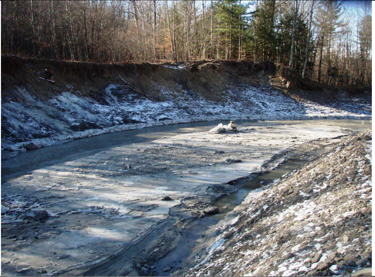
Photo 29: Looking DS at overwidened channel w/ raw banks and little bed armoring
