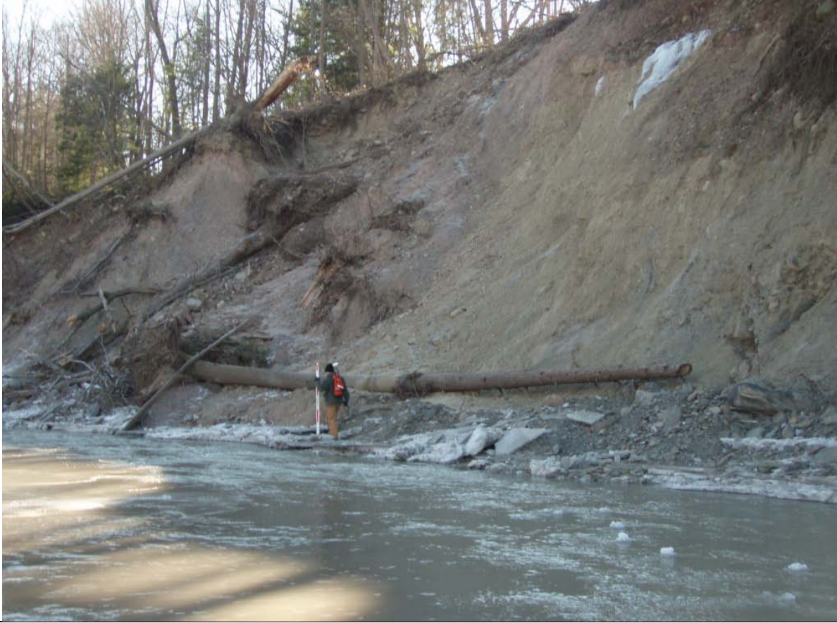
Photo 13: Looking upstream at approx. 40-ft high raw left bank
