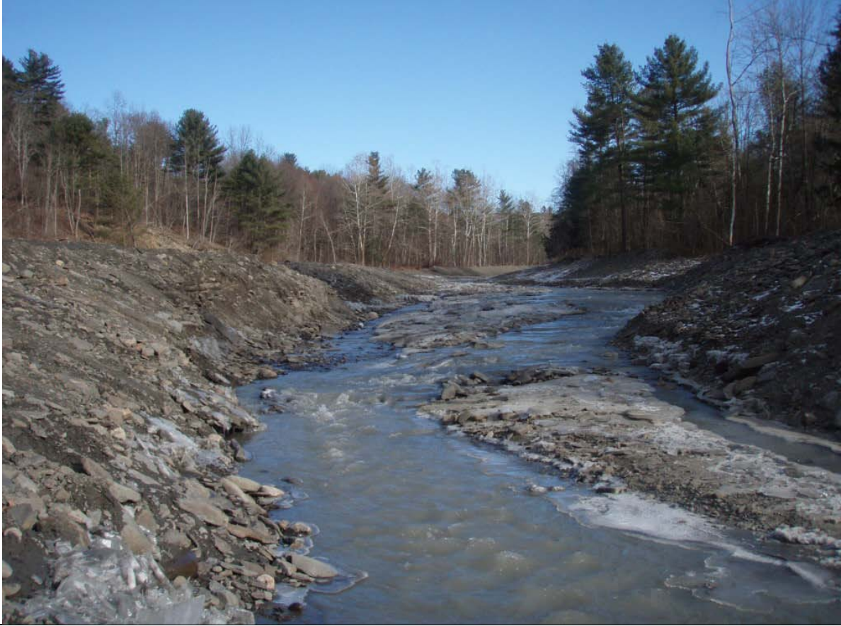
Photo 48: Looking upstream at channel with raw banks
