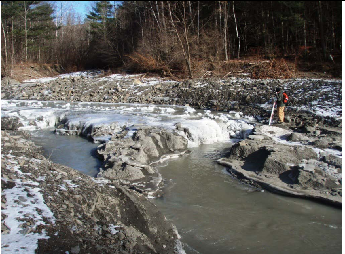
Photo 44: Looking upstream at recent downcutting in exposed clay/silt bed material
