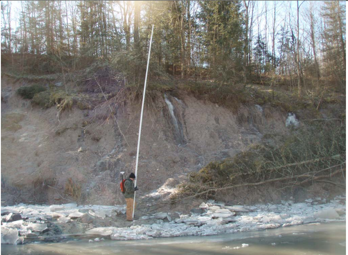
Photo 5: Approx. 26-ft high raw left bank
