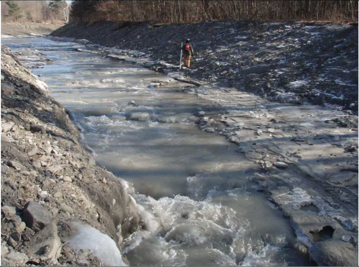
Photo 18: Looking upstream at typical channelized section w/ little bed armoring
