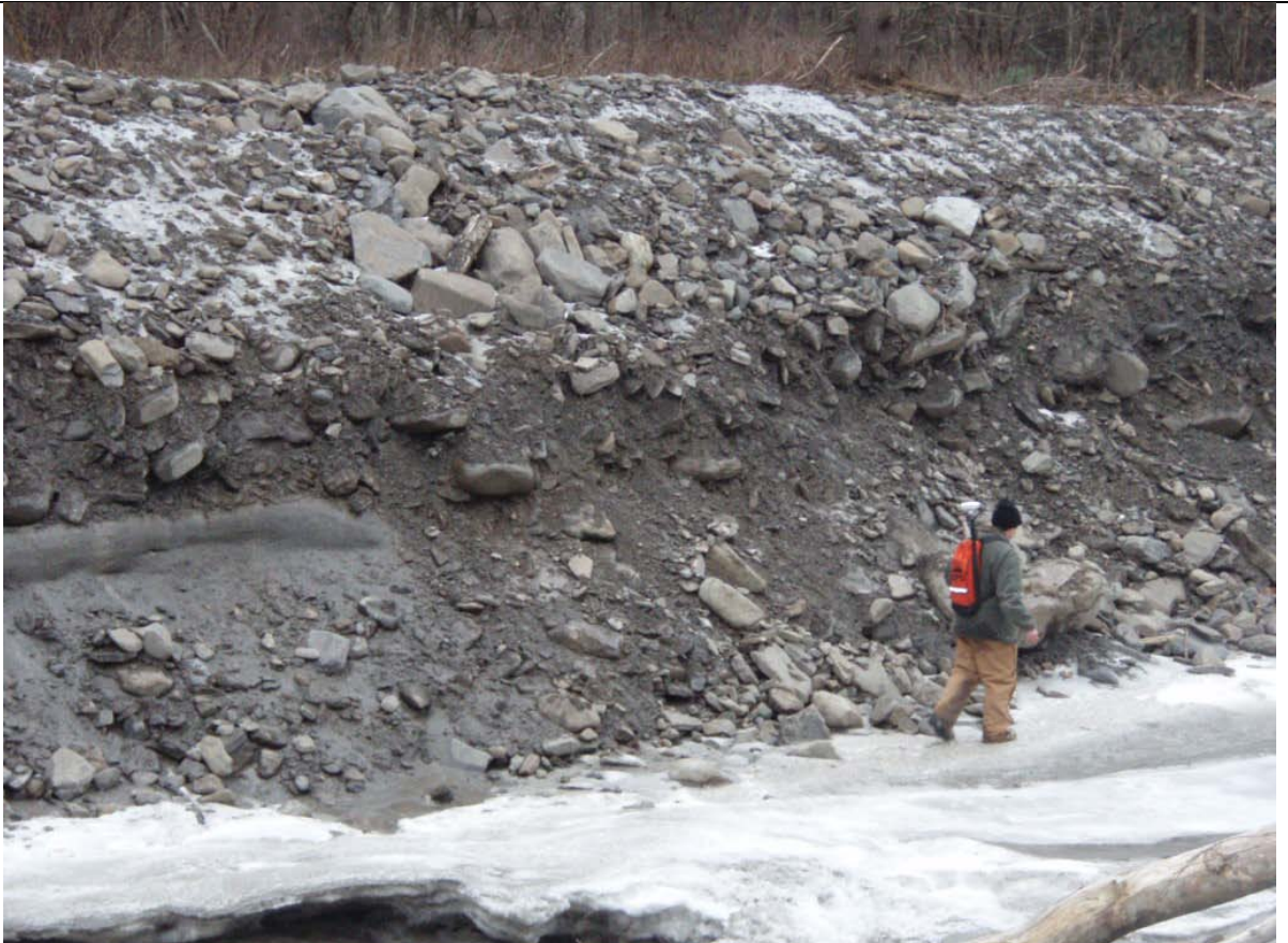
Photo 106 (1/24/12): approx. 20-ft high raw left bank across from sheetpiling nr. Brooky H.
