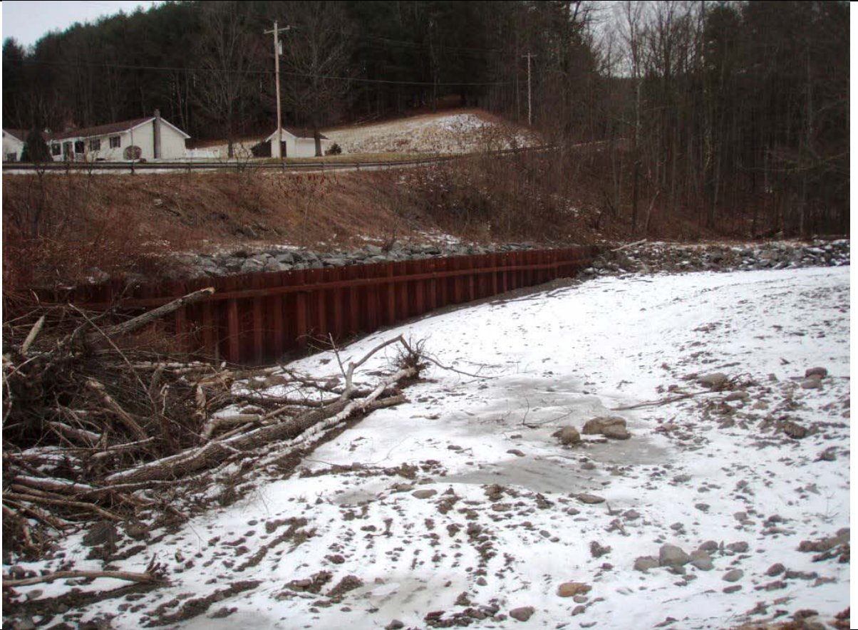
Photo 102: Sheetpiling along Right Bank near Brooky Hollow (original channel alignment?)
