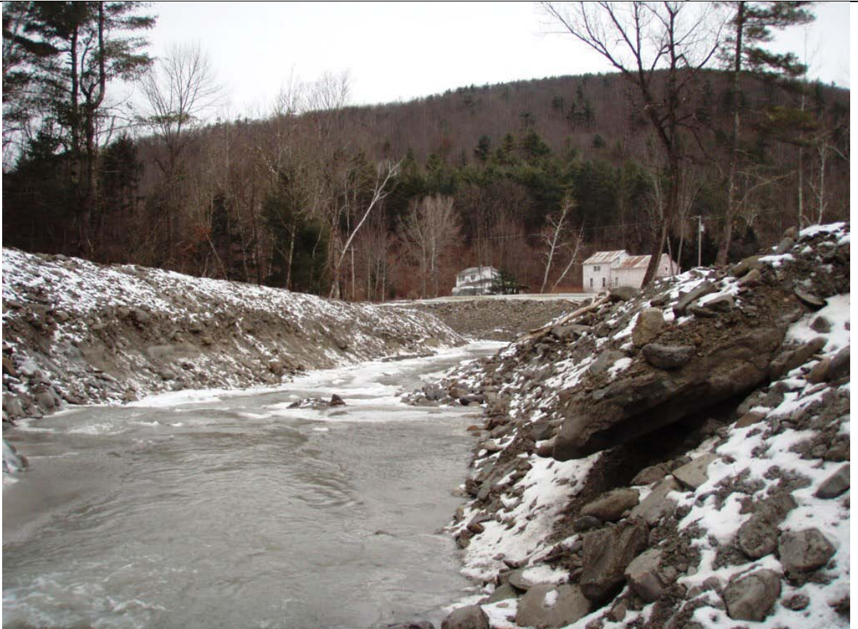
Photo 99 (1/19/12): Looking DS near upper end of reach toward Brooky Hollow
