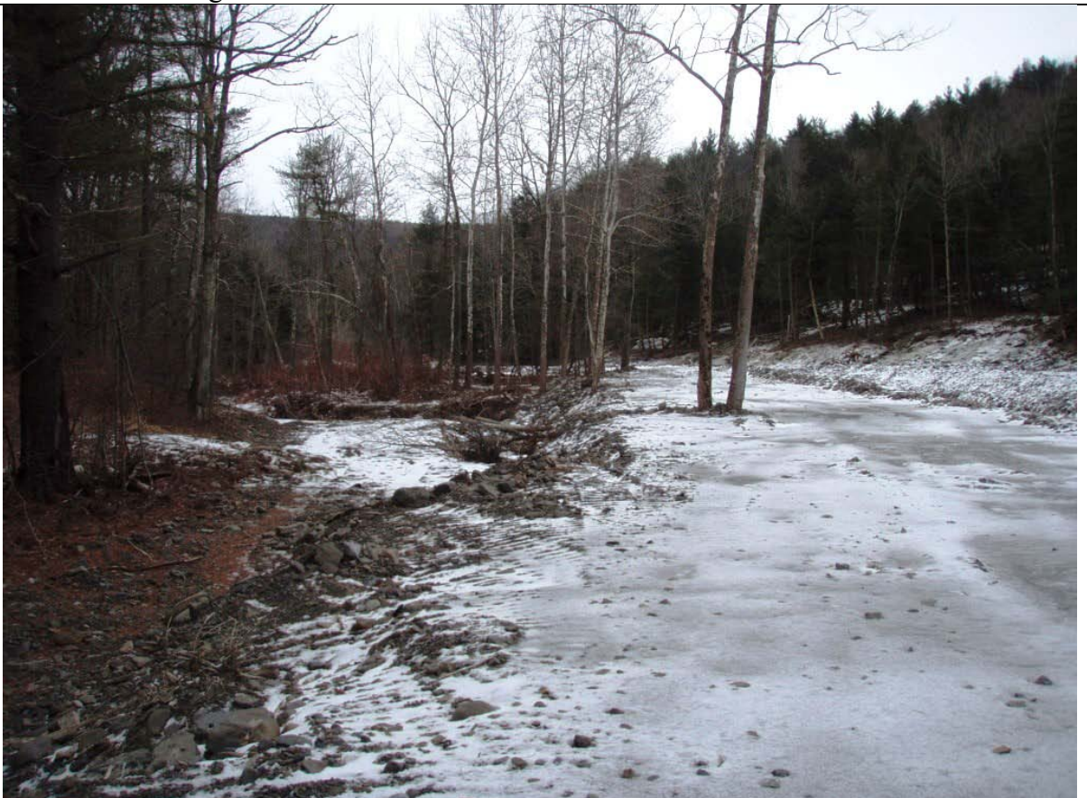
Photo 90: Looking US near mid-reach (possibly remnants of original channel @ left)
