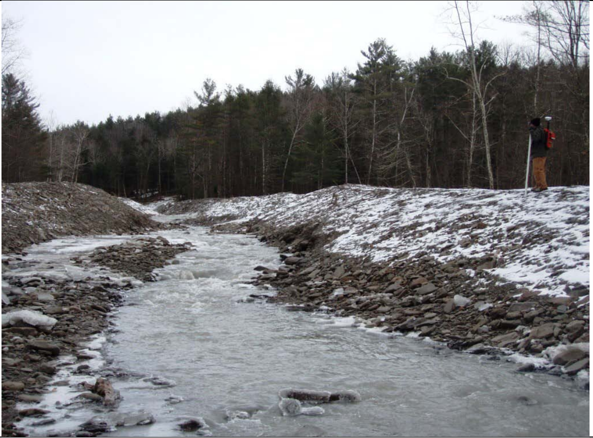
Photo 83: Looking US near mid-reach where old meander bends have been abandoned
