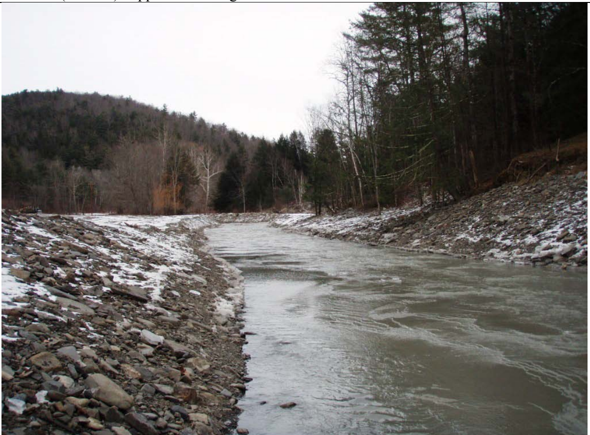
Photo 68 (1/19/12): Looking upstream at lower end of Reach C
