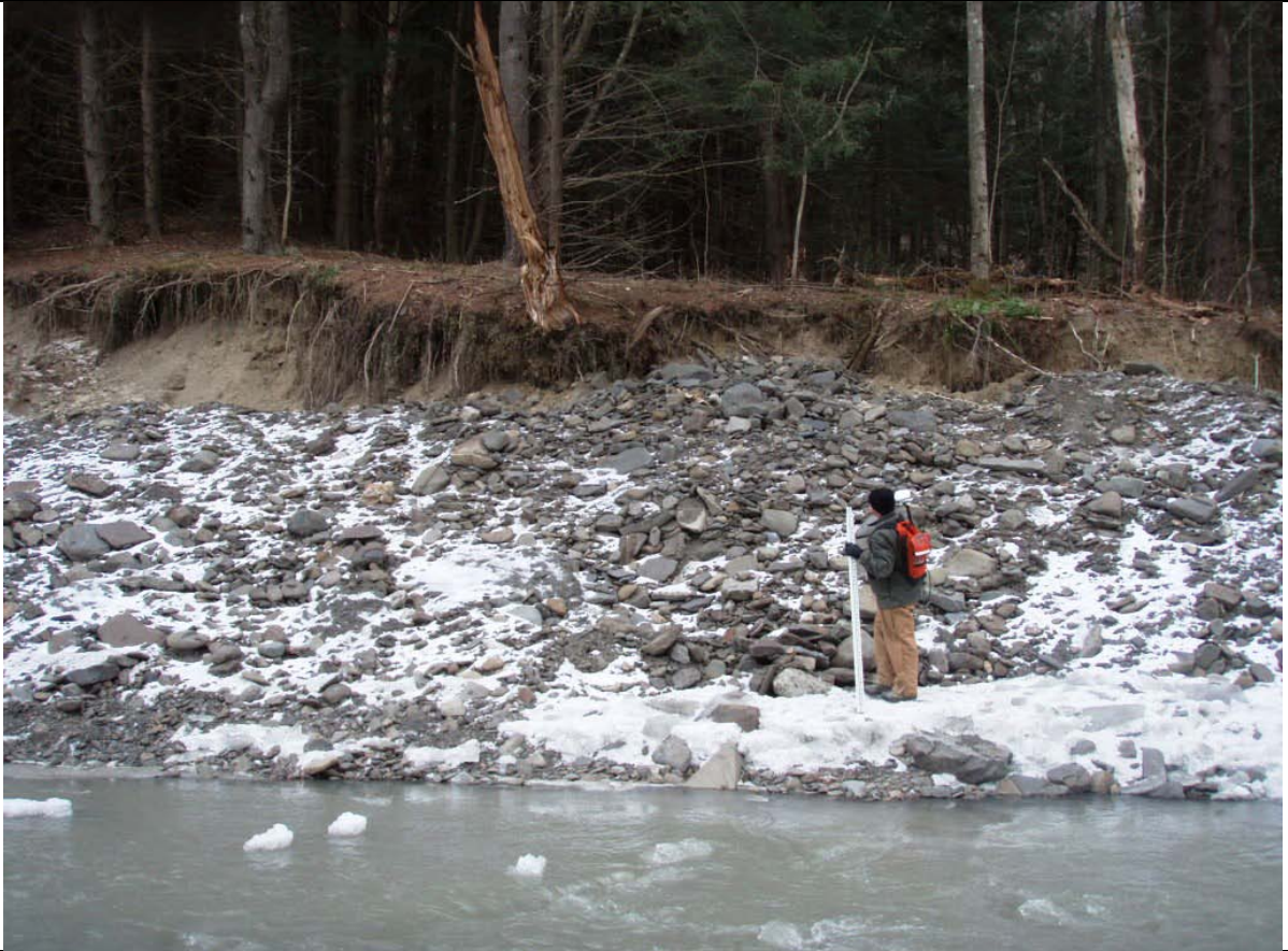
Photo 67 (1/19/12): approx. 18-ft high raw left bank near lower end of Reach C
