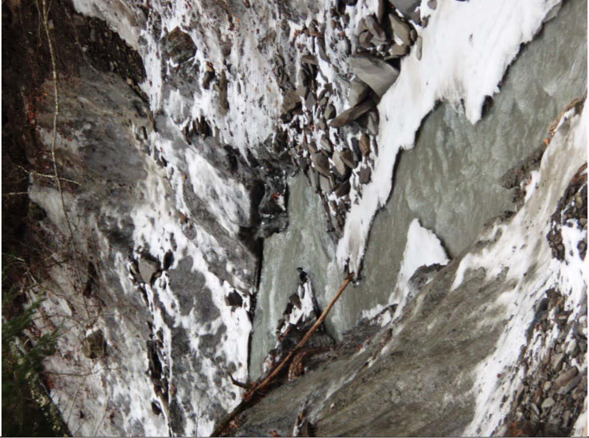
Photo 50: View showing that most bed and lower bank armoring has been washed away
